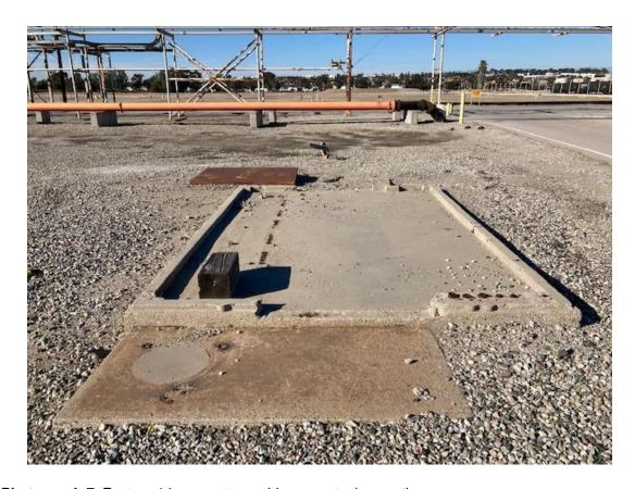
**Photograph 7**. Feature 14, concrete machine mount, view north.
